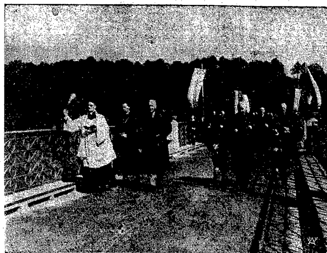
Nowy most na Pilicy.
